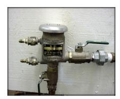
Used mainly on lawn irrigation systems. It has a one way check and a spring loaded air inlet valve that closes when City water main pressure drops.
