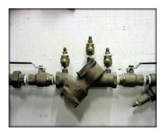
Operates similar to a Pressure Vacuum Breaker. Used on low hazard buildings, for irrigation, and on fire lines.
