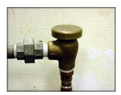
It has an air inlet valve that will drop to draw in air thus preventing customer system water from entering the City's water mains.
