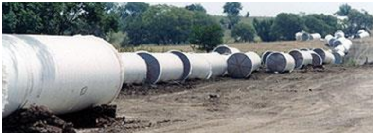
Lake Chapman Pipeline before being placed underground.
