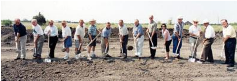
City council and city staff dig-in for the groundbreaking of the Lake Chapman pipeline, 2001.
