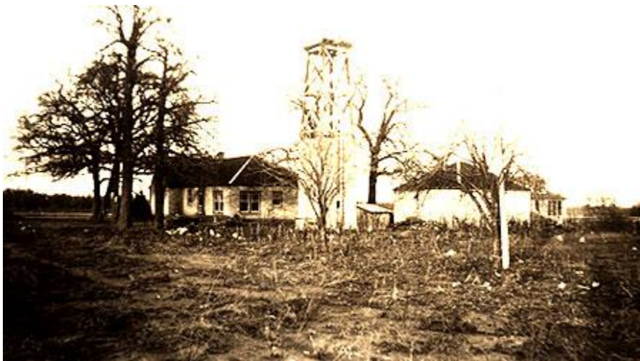
This photo from 1930 shows a house that has a well and water storage tank in the back yard. The house was at the southwest corner of Pioneer Drive and Hawthorne Street.
