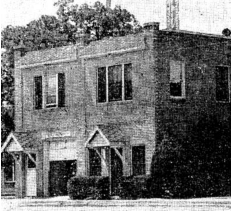
In 1932, the City of Irving joined with the Dallas County Irving Fresh Water Supply District #5 in building the city's first city hall and water district office.
