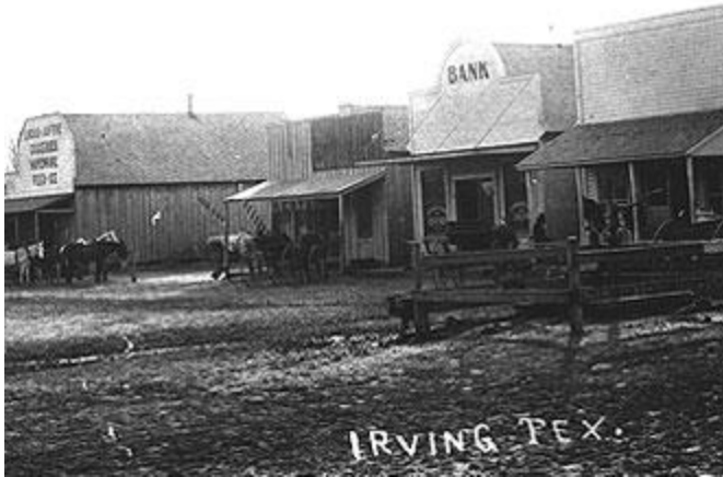
Before the water tower was constructed, the well in the middle of the intersection was operated by a hand-pump. The right side of this photo (1908) shows the well surrounded by a small fence. The pump handle is also visible.
